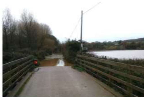
Access along South Farm Road compromised during a flood event
